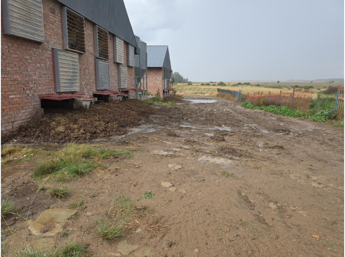
Figure 7: View looking east along the southern elevation of the layer houses. The ground immediately adjacent to the structures is compacted and heavily trafficked; no geological exposures are present. GPS (EXIF): 29.465702°S, 25.995148°E (29°27'56.53"S, 25°59'42.53"E); Field assessment: 5 May 2026; Banzai Environmental).
